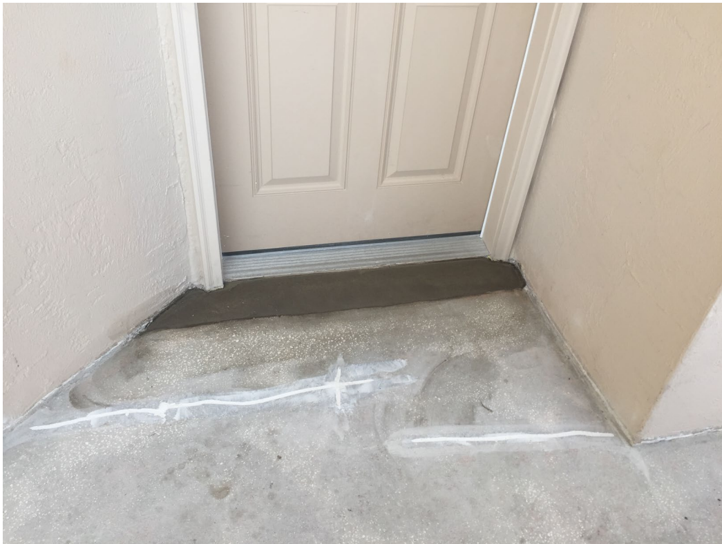
Picture 2: Typical new unit entry door topping
