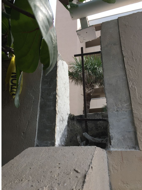
Picture 1: Completed wall excavation
